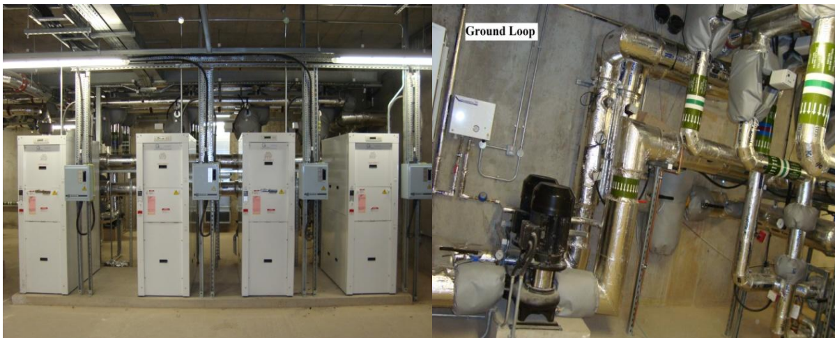
Fig.3. The Heat Pump Installation
