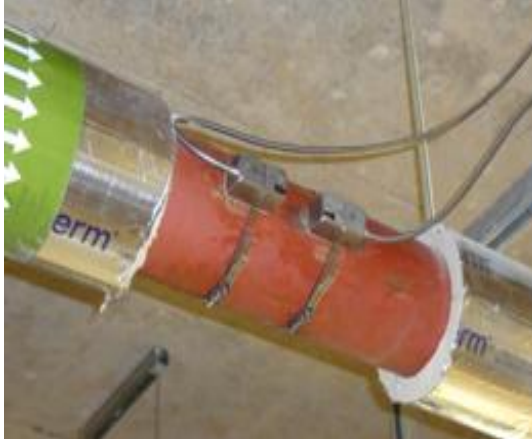
Fig.8 Ultrasonic Flow meter Sensor
