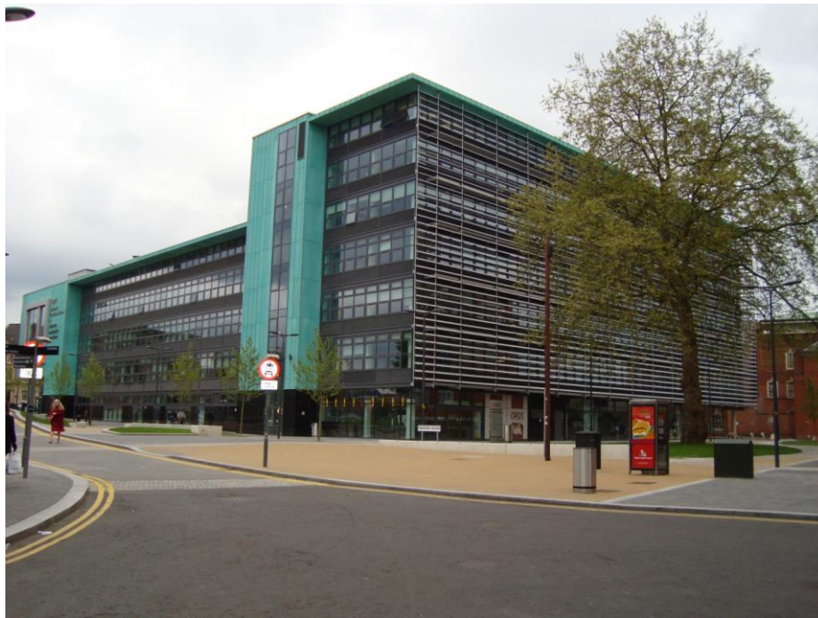
Fig.1. The North Western elevation of the Hugh Aston Building at DMU
